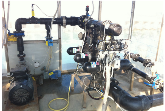
Portoverde filtration system
